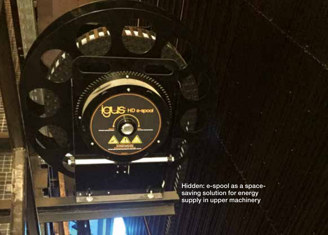
The energy reaches the stage quietly, lubrication and maintenance-free
