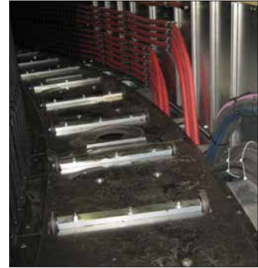
Rotary system with “floating islands” for safe operation on rough seas – rotation angle 540°
